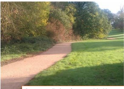
An unmetalled surface provided in Enfield. This performed well despite flooding during extreme weather conditions but areas with a significant gradient and high surface water run-off suffered, which may be an issue for the bridleway.
